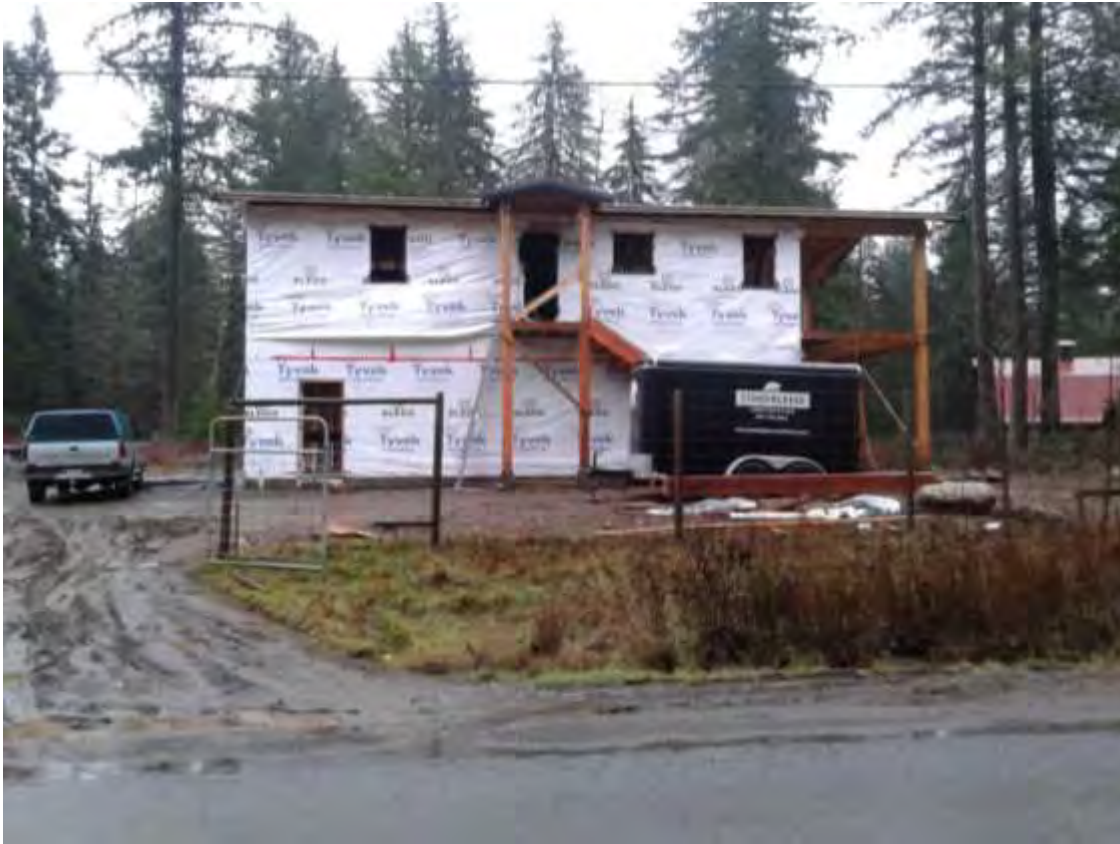
Figure 3: Photo of Unfinished Carriage House as Seen from Railway Avenue
